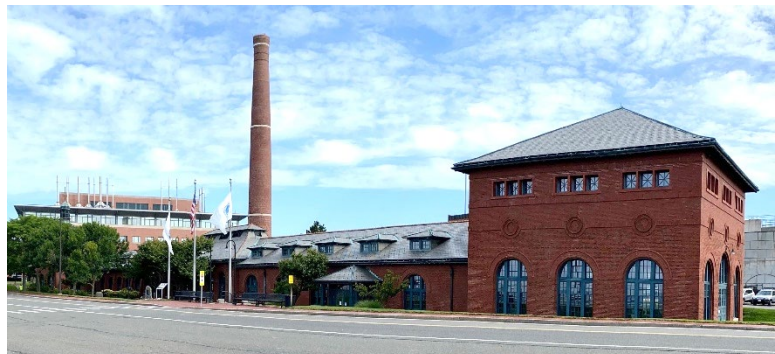
Deer Island Historic Pump Station
